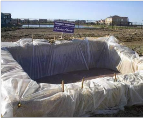
Plate 3-1 Typical concrete wash out areas
