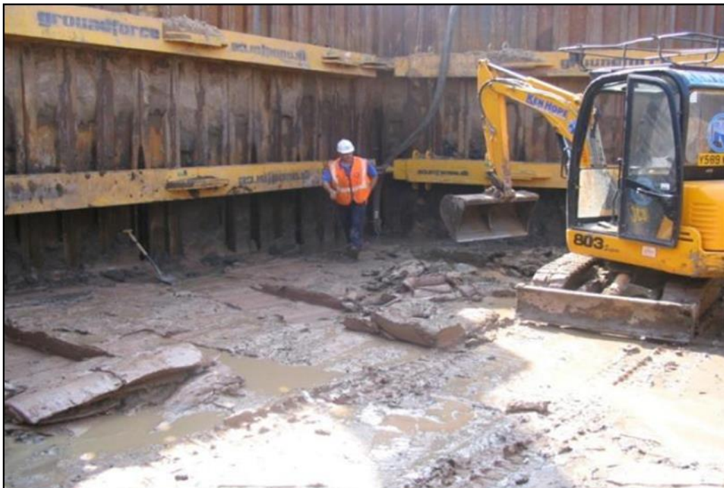
Plate 4.10 Sheet piling a hardstand in Cumbria, UK
