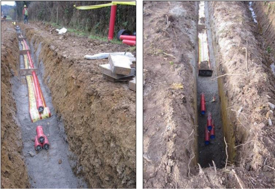
Plate 2-1 View of concrete cover in cable trench
