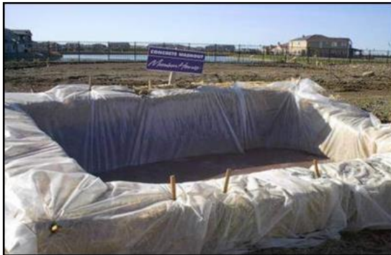
Plate 4.6 Concrete washout area
