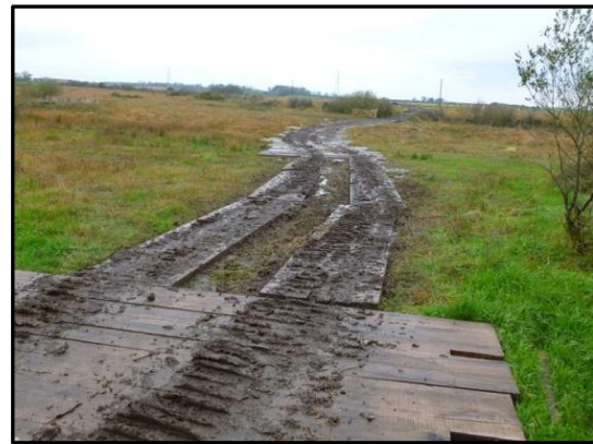
Plate 4.5 Bog mat protecting ground by excavator.
