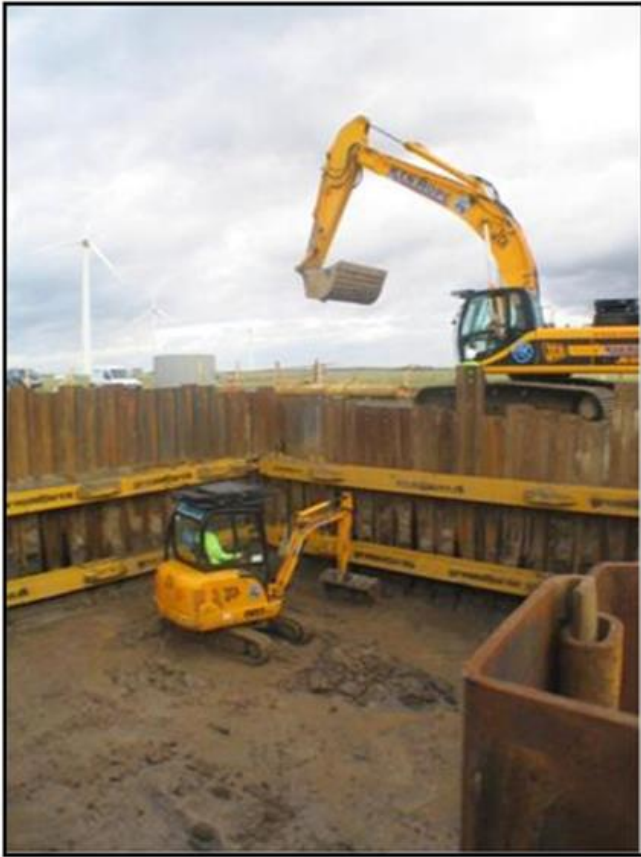
Plate 4.9 Sheet piling a hardstand in Cumbria, UK
