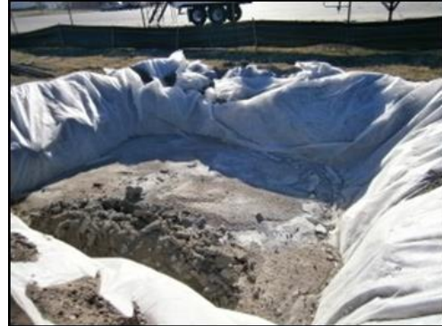
Plate 4.7 Concrete washout area
