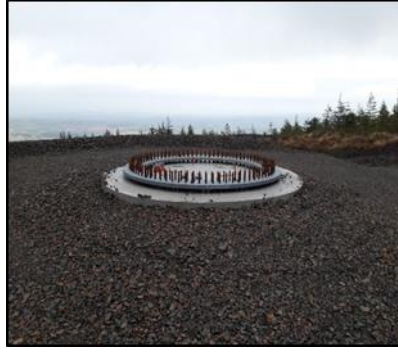
Plate 4.3 Steel reinforcement being added
