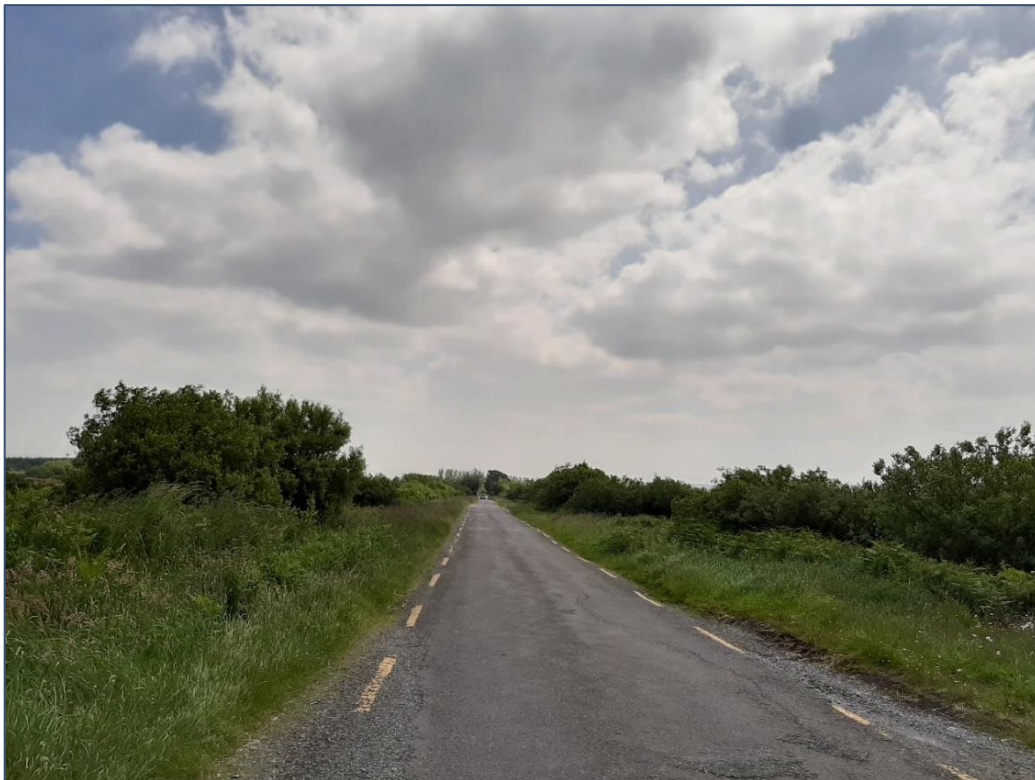
Plate 6- 11 Made roadway within the site study boundary classified as buildings and artificial surfaces (BL3)
