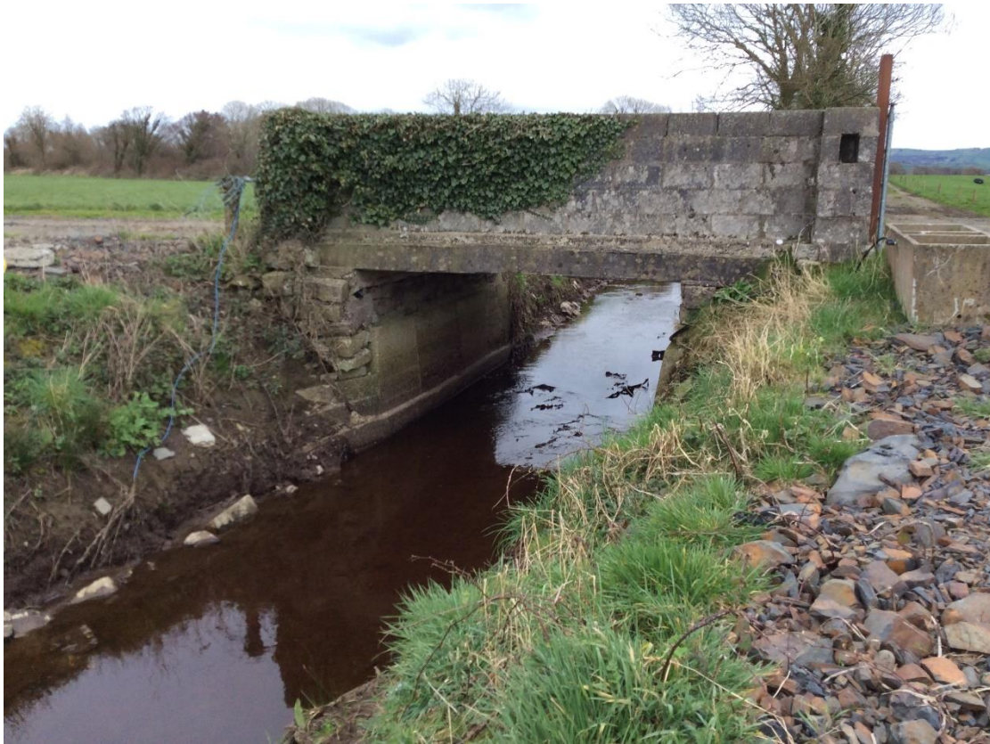
Plate 12.12: CH9 Poulboy Bridge, looking SE.
