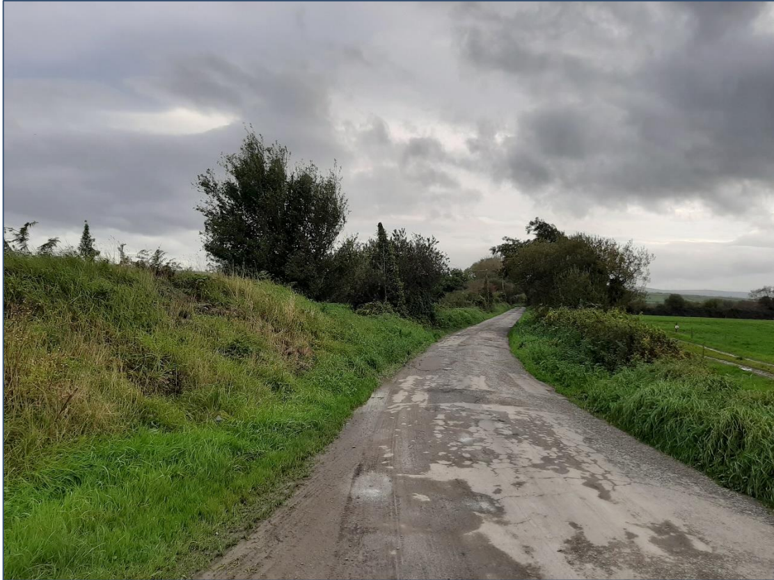
Plate 6- 31 Location 6 – Existing roadway boarded by Earth bank
