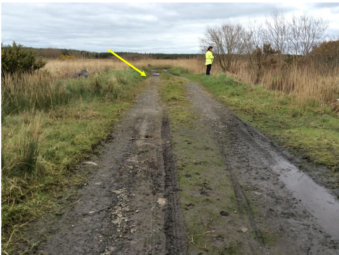
Plate 12.7: Low rise of KE009-088 where it is traversed by an existing track within the bog, looking NE.
