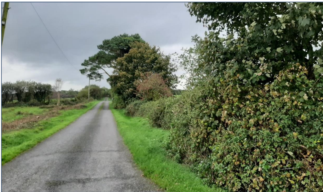
Plate 6- 27 Location 4 – Existing roadway bordered by Hedgerow
