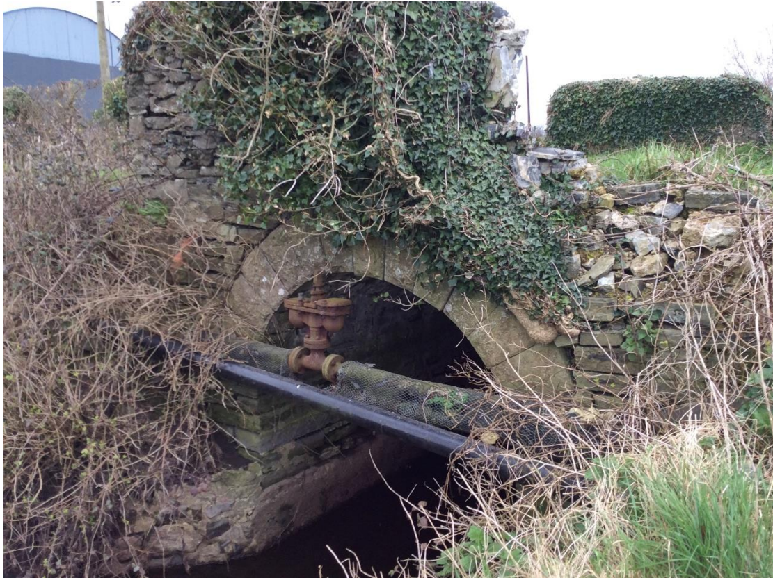
Plate 12.13: CH10 MacElligot's Bridge, looking SE.
