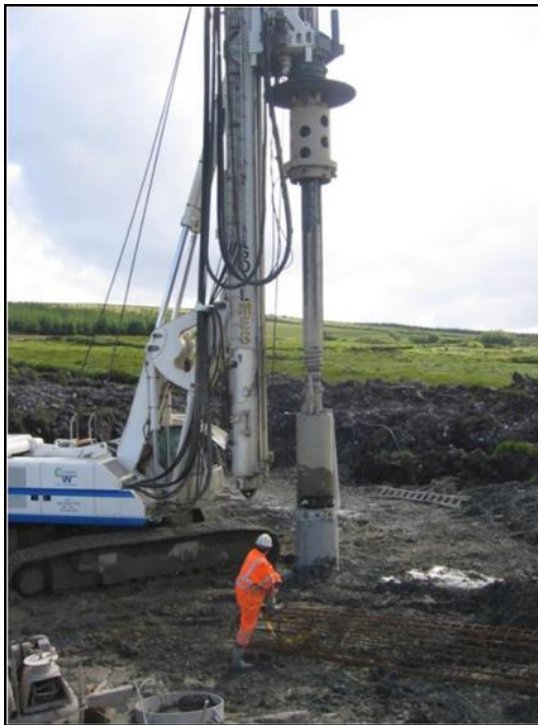
Plate 4.8 Piling Rig on a piling platform at a turbine foundation
