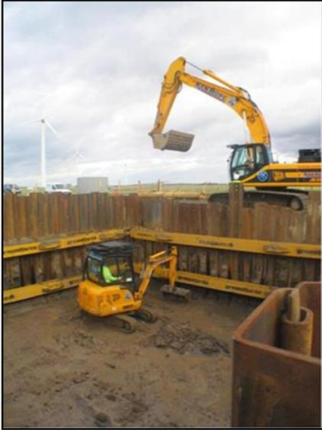
Plate 4.9 Sheet piling a hardstand in Cumbria, UK
