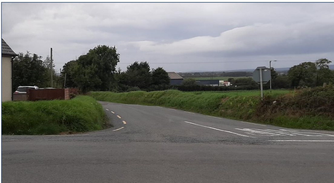
Plate 6- 25 Location 2 – Existing roadway across road junction boarded by Earth bank
