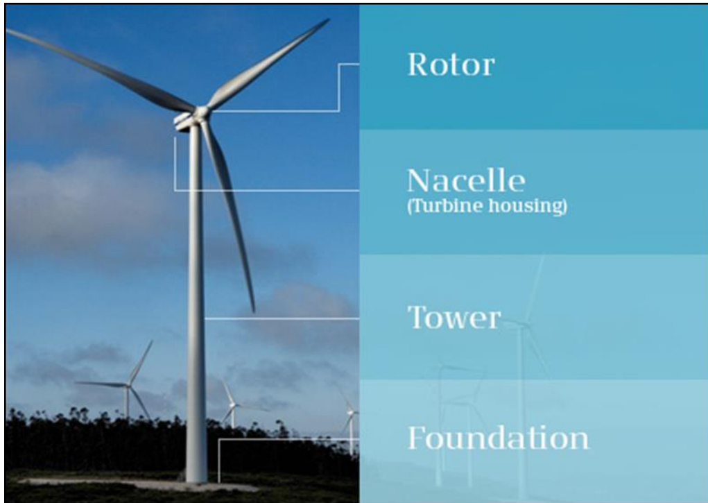
Plate 4.1 Wind turbine components
