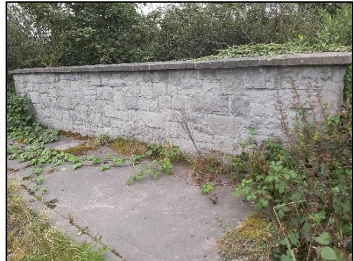
Plate 6- 46 Bridge structure at Pallas watercourse
