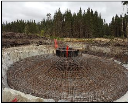
Plate 4.2 Levelled turbine tower ‘can’
