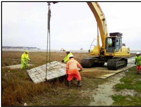
Plate 4.4 Bog mat being laid in position by excavator
